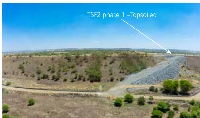
TSF 2 phase 1 – Topsoil and revegetation in progress
