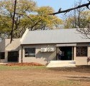
Arxo Metals Renewable Energy Centre
