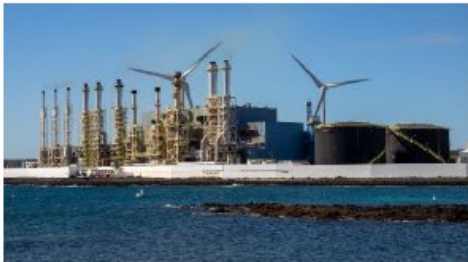
Seawater Desalination Plants
